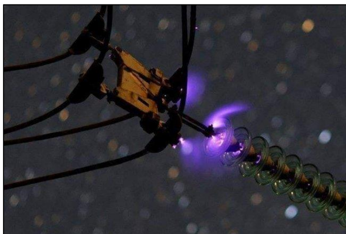
Figure. 1. Corona discharge occurring on an insulator in a high-voltage overhead power transmission line with a voltage of more than 500 kV
