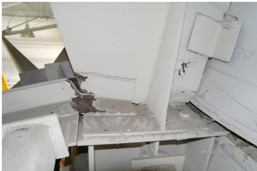
Fig. 11: Brittle fracture of lower chord
