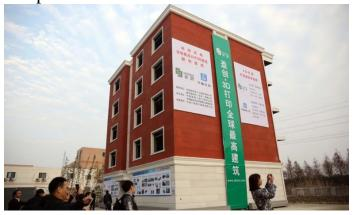
The WinSun buildings were created using a custom-made giant printer, measuring 6.6 meters wide by 10 meters tall that took the company 12 years to develop. Printing horizontal layers of "ink" – a mixture of glass fiber, steel, cement, hardening agents and recycled construction waste – the machine creates several
